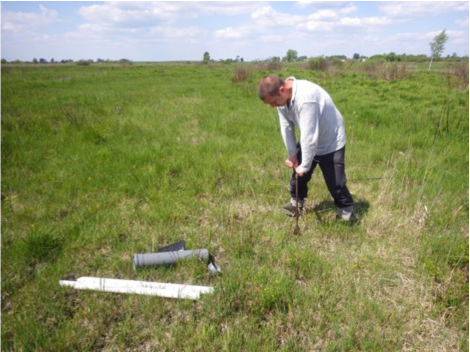
Photo 129: Installation of a piezometer with a measuring device (photo by E. Gutowska).
