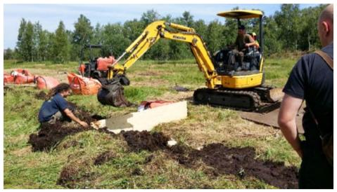
Photo 89. Works carried out to block water outflow in drainage ditches. Solid wooden walls are driven into the peat bed and the ditches are filled with sawdust and covered with peat (photo D. Horabik).
