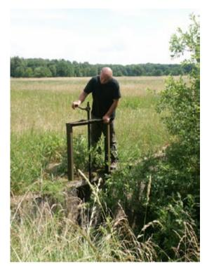
Photo 55: Concrete gate with adjustable damming by means of a metal plate (photo B. Utracka-Minko).
