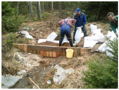
Photo 96. Blocking of the ditch by construction of 2 tight partitions filled with clay and with local peat on top (source: http://www.kp.org.pl/plbaltbogs/)
