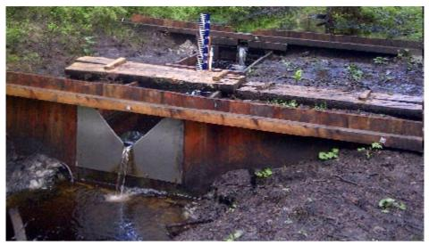
Photo 83. A damming barrier with V-shaped metal overflow (photo M. Makles).
