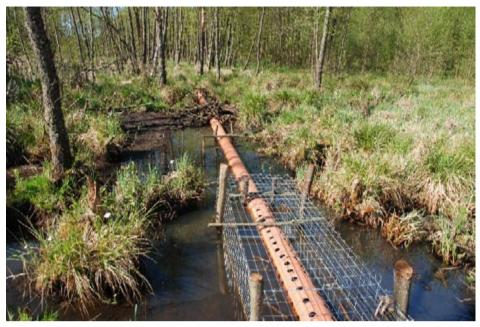
Photo 59: Cases of negative, excessive flooding of fens by beavers can be limited by special pipes inserted into the dams. "Cooperation" with beavers in fen protection is much cheaper and does not require laborious, often completely unnecessary, legal procedures (photo R. Stańko).
