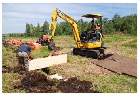
Photo 54: A plywood partition is pressed into the fen into a gap (previously made by means of a thick metal sheet driven in and pulled out by an excavator) by means of a small excavator. Bags filled with sawdust (seen in the background) are intended to fill the ditch sections between the gates. Fen in the Franche-Comté region in Jura, France (cf., also chapter 7; photo R. Stańko).
