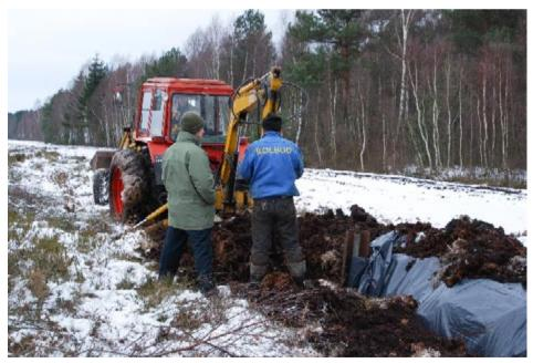
Photo 57: Installation of plastic foil on the edges of the fen in order to limit its drainage by a neighboring drainage ditch (photo R. Stańko).
