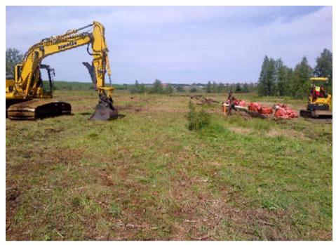
Photo 90. After completion of the filling works, the surface was additionally compacted using heavy equipment (photo M. Makles).
