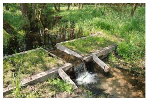
Photo 53: A wooden partition made of two watertight walls with filling; perfect for ditches and watercourses with significant water flow (the Mielęcin-Bukowo site in the Drawa Forest, photo R. Stańko).
