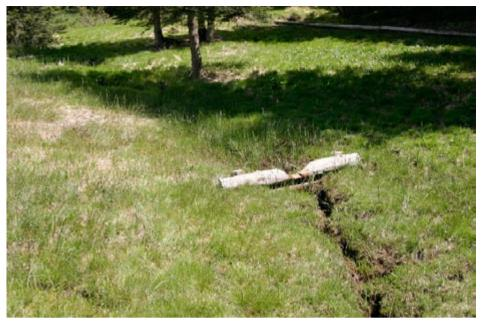
Photo 95. A damming barrier constructed under the project (photo D. Horabik).
