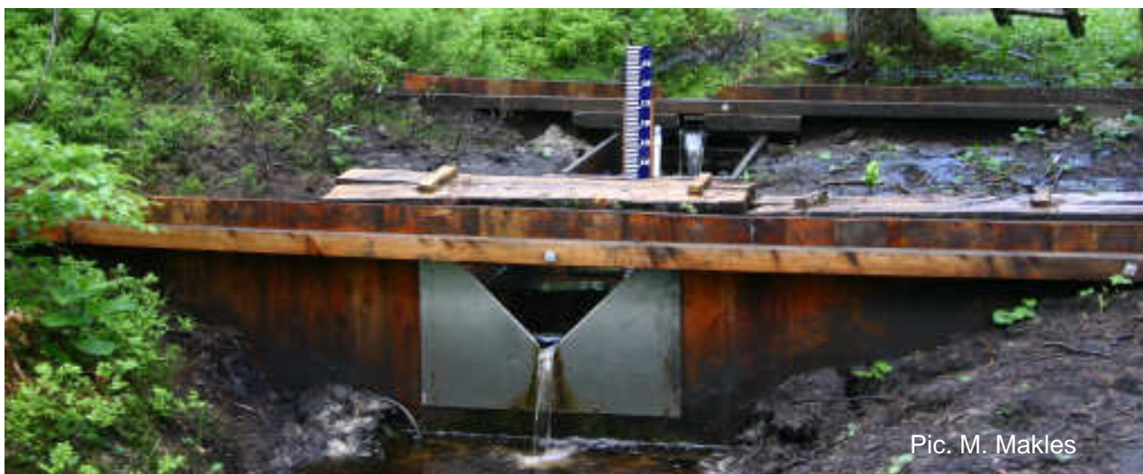
Pic. 28. Water gate with a V-shaped metal gate.
