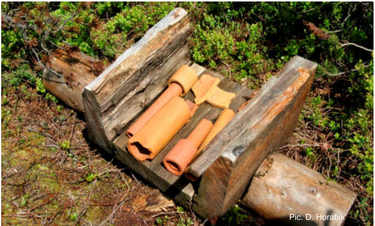
Pic. 25. Wood filling of the channel and also the ceramic elements of the drainage system
