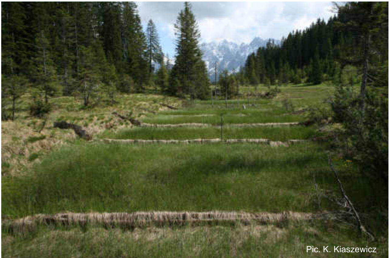
Pic. 29. Baffles slowing down the runoff have almost completely blended in with the landscape.
